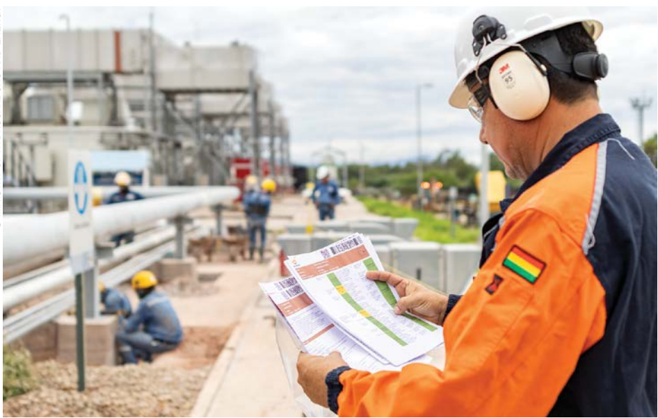
Change is coming as Bolivia's hydrocarbons and mining sectors seek revival.
